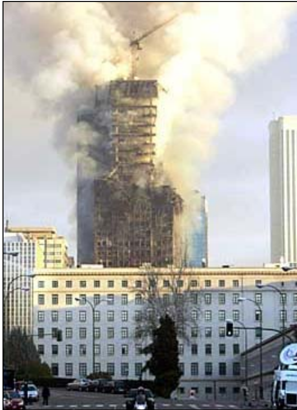
Windsor Building during the fire
