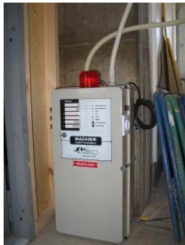
Air sampling construction site fire alarm – MADAMM
